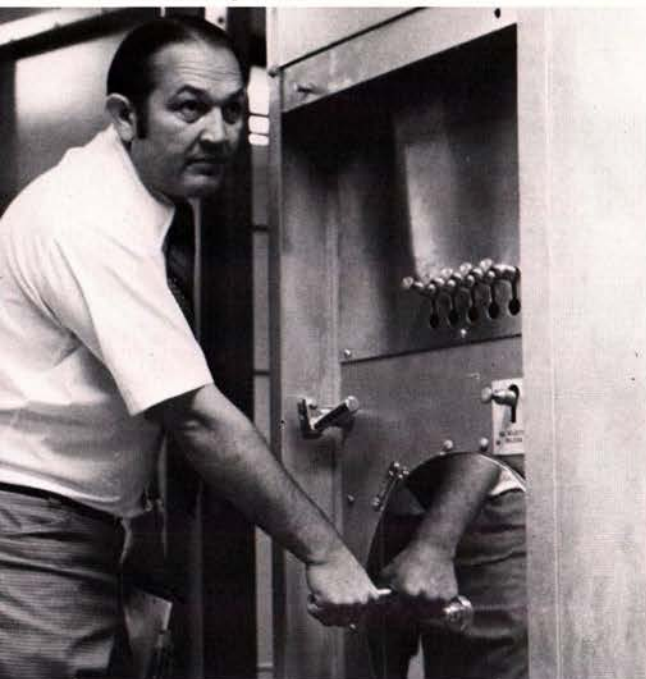
Sheriff Newmans demonstrates controls that allow jailers to open and close cell doors without entering the cell block.
